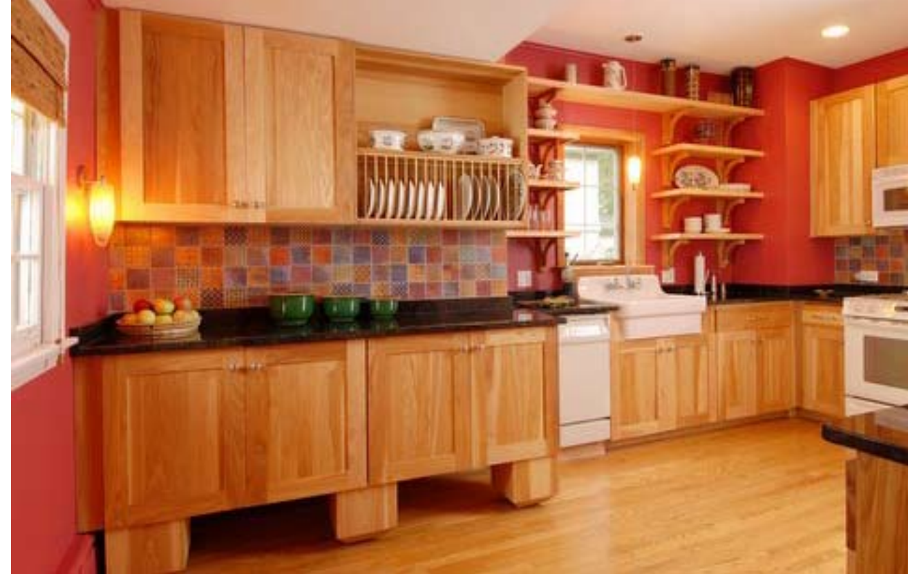
At left is a custom kitchen by Whitney Wood Works with all wood hickory doors and an all natural oil finish. Boxes are of Columbia PureBond plywood and drawer boxes of highly sustainable German beech.
